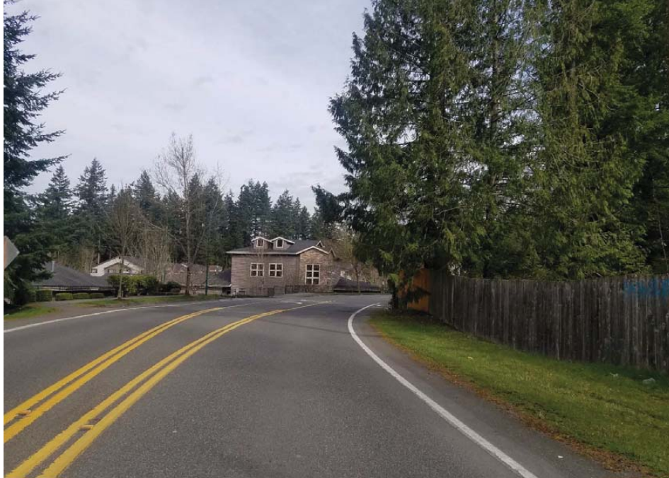
View from North Creek Drive headed northwest
