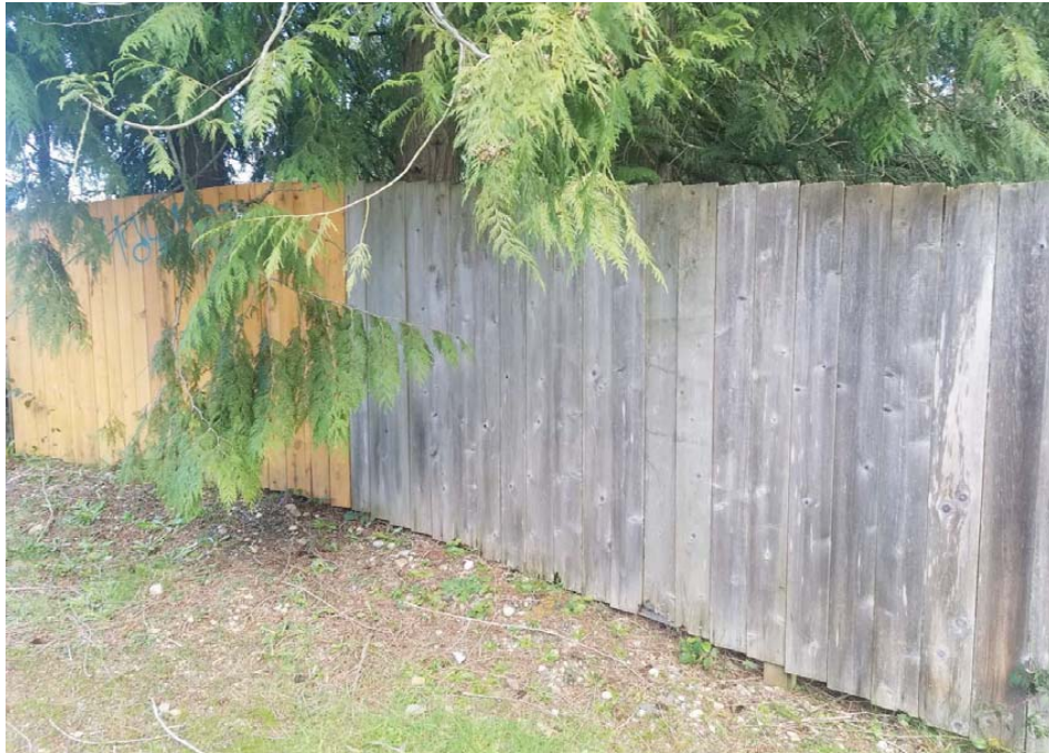
Existing fence along North Creek Drive.
